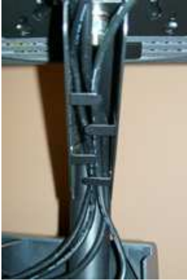
Figure 11, Monitor Arm Cables
